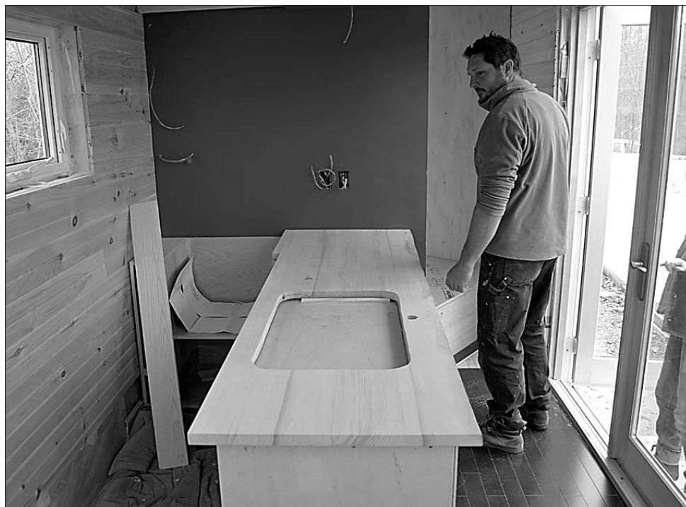
Jamie Constable peruses what will be the Tiny Shelter's kitchen area.
